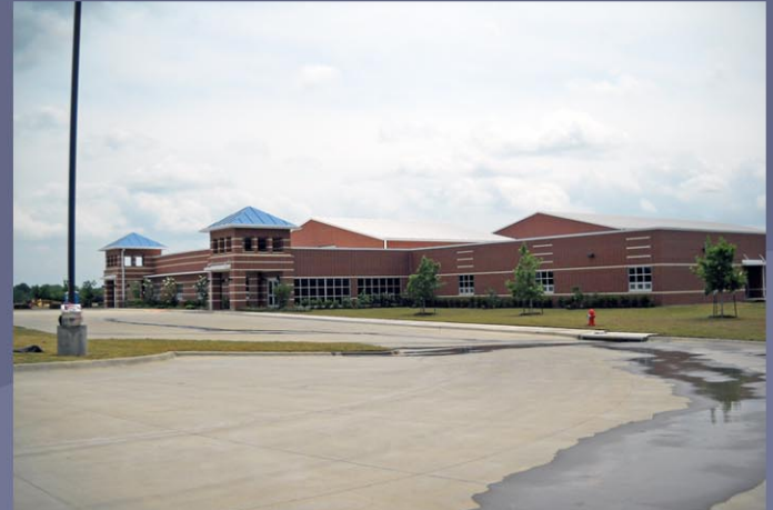
The landscaping around the building has been installed. Here is looking at the front entry.
